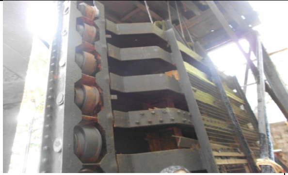
DAMAGED GUIDE ROLLERS OF INTER CONNECTING TUNNEL GATE
